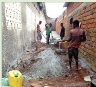
LUOZI LAGERE SCHOOL: Afwateringswerken
